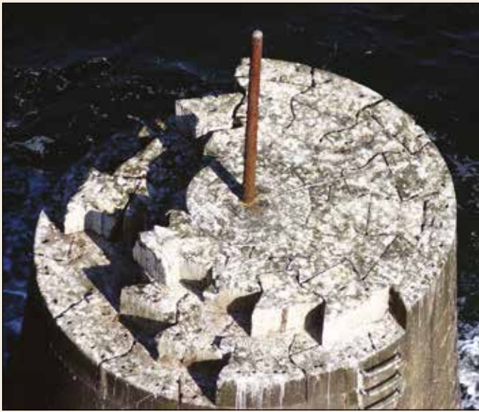
A remarkable view showing the damage over a century of winter storms have done to what remains of Smeaton's Eddystone. The dovetailed blocks, trenail holes and even a couple of marble joggles are clearly visible. This image was taken a few years ago; today the damage is much worse. How long before the sea reclaims this historic monument? Photo by John Nicholls
